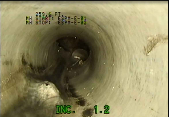
EXISTING CONDITIONS AT STA. 5+33.5
