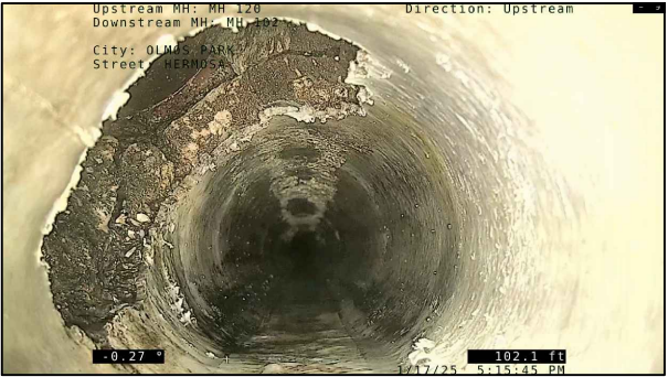
EXISTING CONDITIONS AT STA. 1+02
