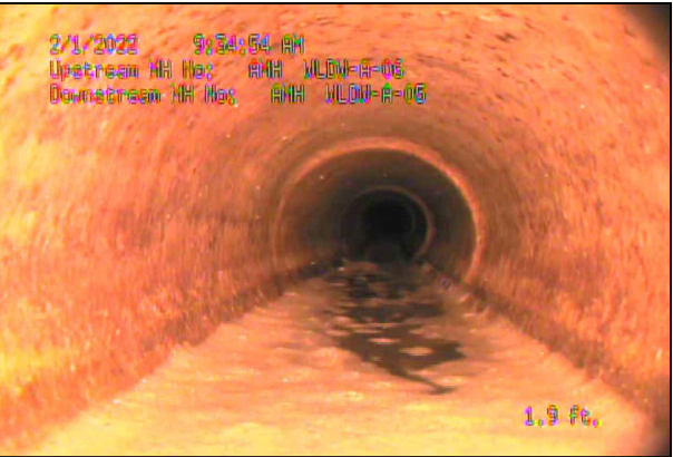
EXISTING CONDITIONS AT STA. 0+02 to STA. 0+07
