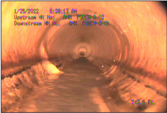
EXISTING CONDITIONS AT STA. 01+82
